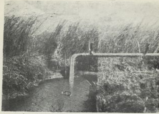
A.—SIPHONING A LARGE POND IN A CUP-LIKE DEPRESSION AMONG THE HILLS.
