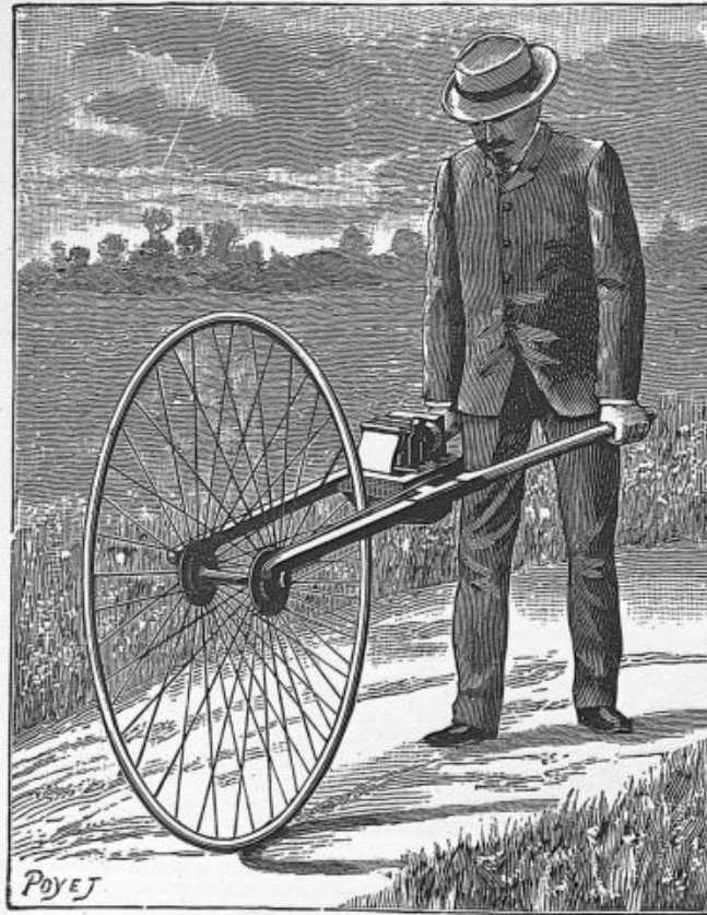
FIG. 30.—Pedestrian pushing an odograph in front of him.
