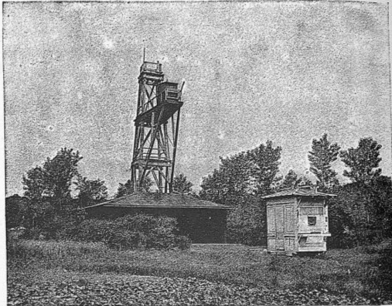
FIG. 49.—Arrangement of the dark background at the Physiological Station. In front of it there is a small chamber running on rails for keeping the apparatus. Above the dark background a framework is arranged for holding the camera at a distance of 12 metres, when it is necessary to photograph from above.
